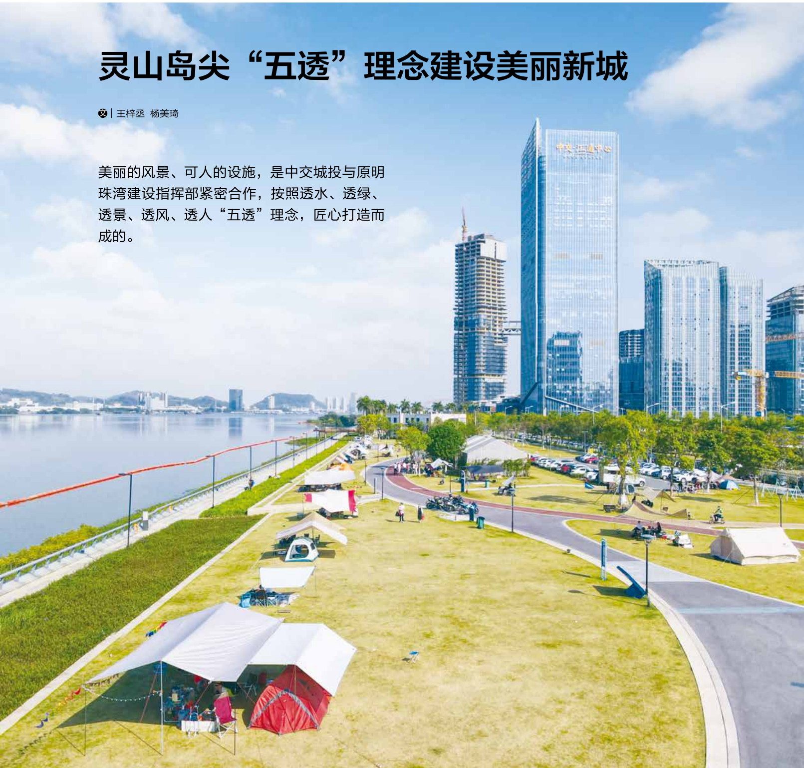
广州南沙灵山岛尖超级堤
